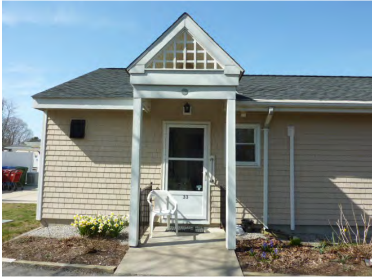
Typical unit front entrance. Concrete stoop with gabled roof, new vinyl siding, new black kitchen exhaust vent, new window, light over entry door, and screen doors that do not latch properly.
