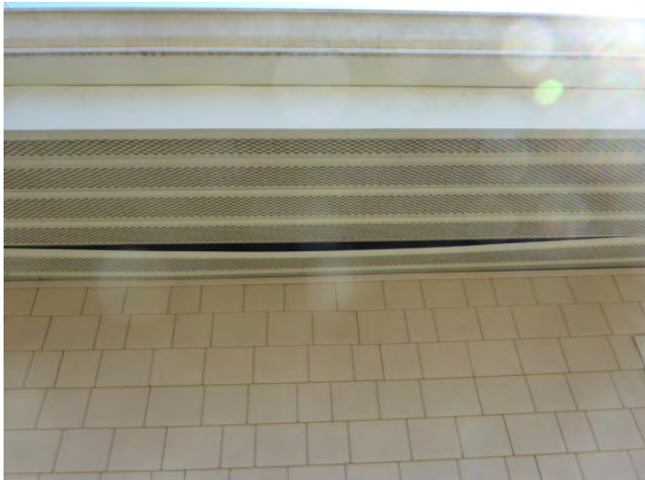
Vinyl soffit failure should be repaired periodically through the term.
