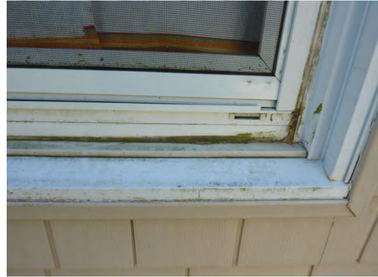
Sealant at new windows typically exhibits organic growth and should be removed and replaced.
