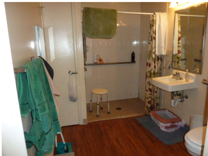
Typical bathroom in 4 designated accessible 1-bedroom apartments has roll in shower. Tile surround is original and shown to be replaced.
