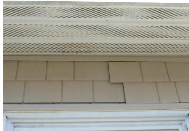
Vinyl siding failures should be repaired periodically through the term.
